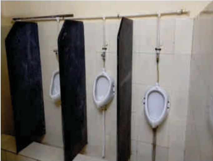
Renovation of Toilets ) Urinals-Dayanand Vedic School-Mulund
