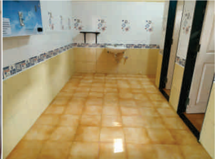
Renovation of Toilets & Urinals-Adarsh Nagar BMC School-Worli
