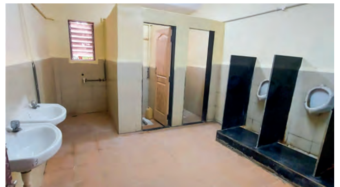
Toilet renovation in Motilal Nagar School, Goregaon West - Mumbai
